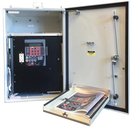
Figure 6-6 M-2979 Recloser Cabinet Internal
